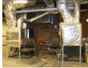
Illustration 14: Water-to-Air Heat pumps in meetinghouse basement
