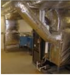
Illustration 14: Water-to-Air Heat pumps in meetinghouse basement
