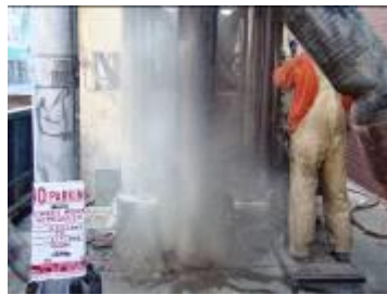
Releasing pressure in bore hole
