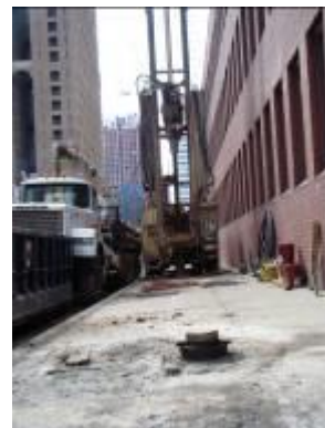
Capped well awaiting next phase
