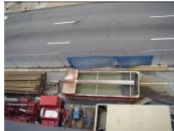
Flatbed with rods Dumpster for tailings
