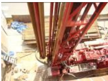
Illustration 6: Air rotary drill rig, two views
