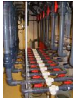
Finished piping and valving system
